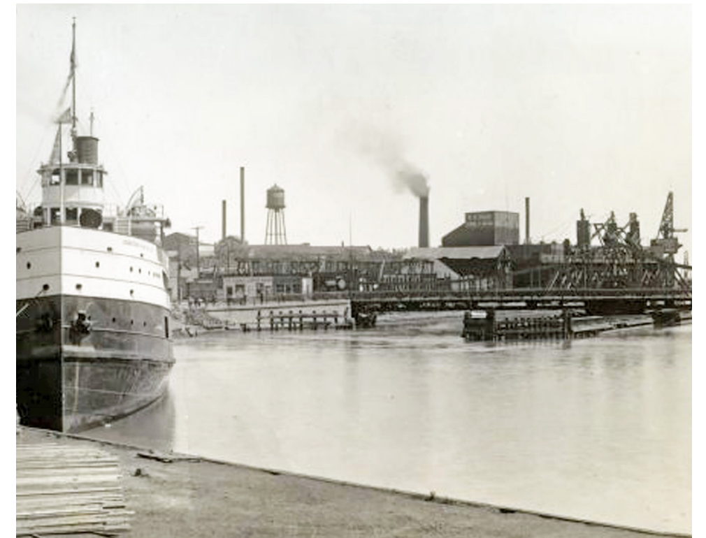
View of Main Street bridge from the West, circa 1910.
