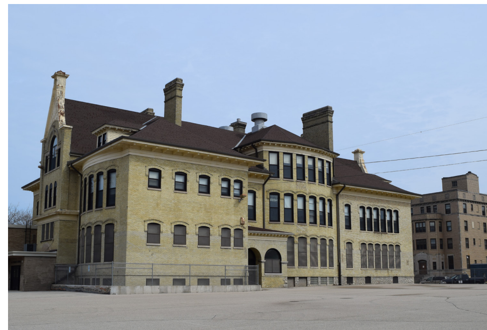
Closed Winslow Elementary School 1325 Park Avenue.
