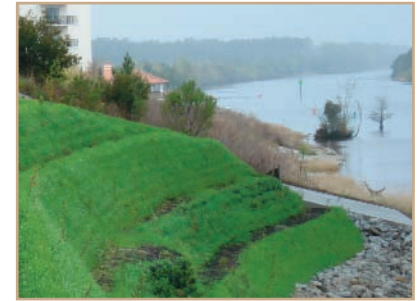
Another option to managing steep slopes or bluffs are living walls which offer eco-friendly erosion protection. A living wall is a vertical arrangement of vegetation that can help infiltrate stormwater runoff and prevent the soil from eroding. Photo courtesy of the Bruce Company.
