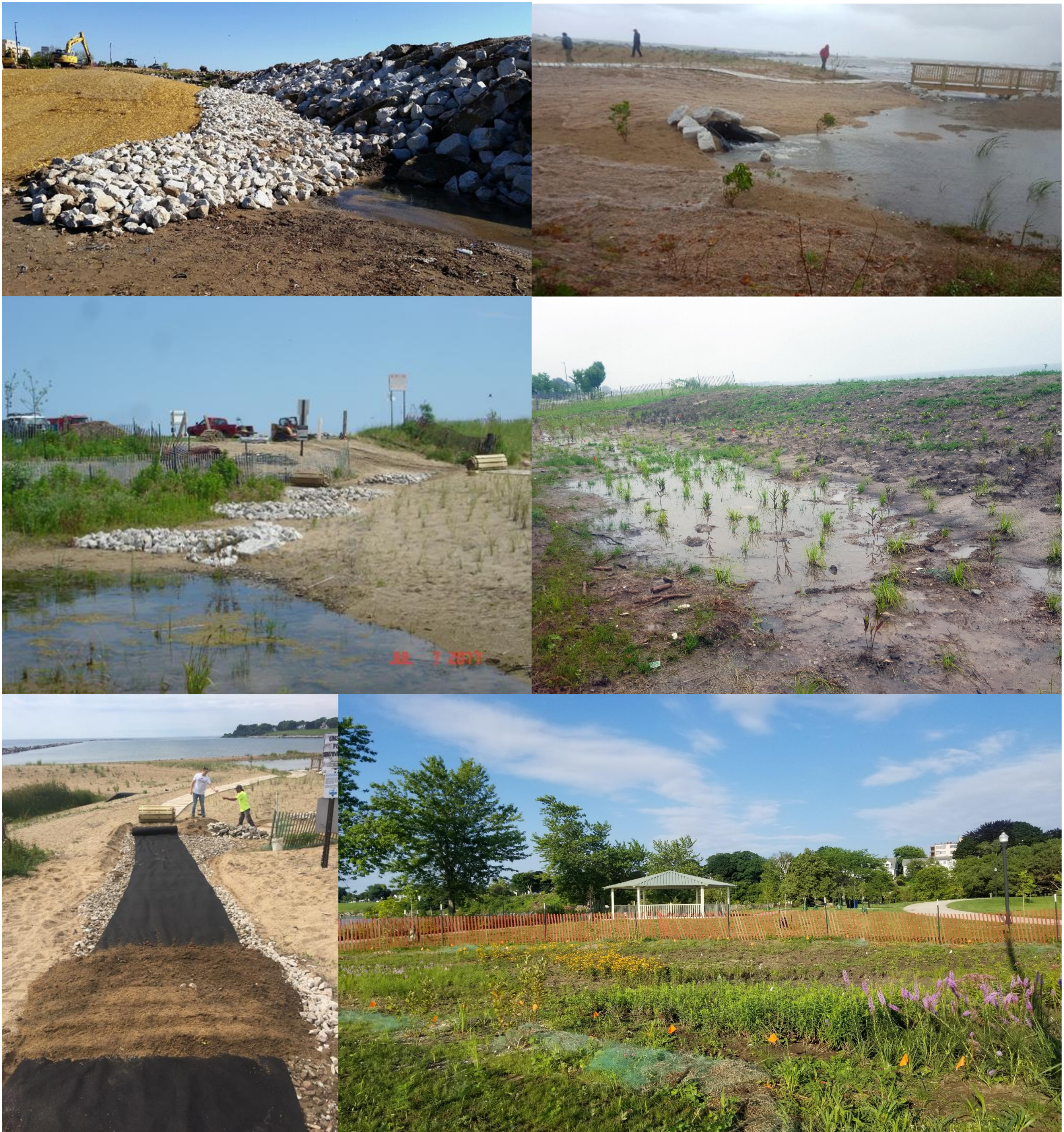
Figure 4. Examples of coastal resiliency measures – Samuel Myers Park (Clockwise from top left: return flow channel, culvert, bioswale, rain garden, French drain and energy dissipators).
