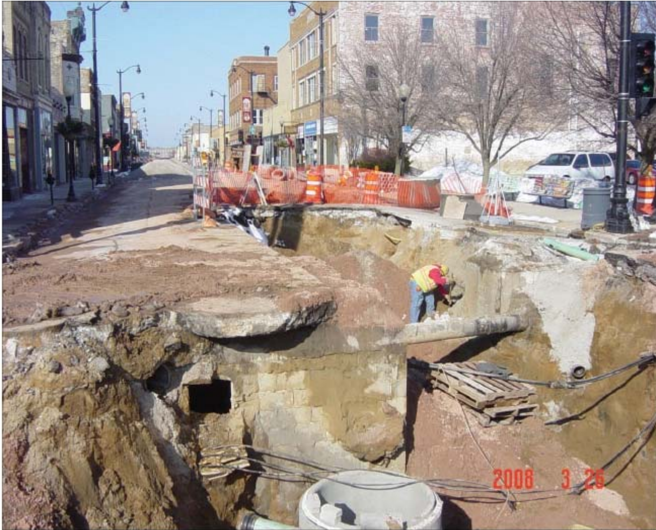
Sewer work in the 400 Block of Sixth Street
