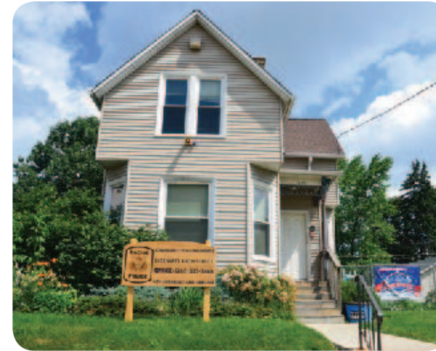
West Sixth Street COP House 1522 W. Sixth Street
