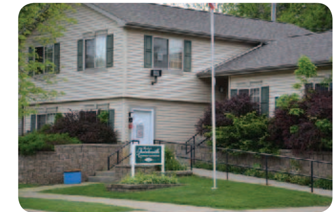
Robert Quintanilla COP House 1140 Geneva Street King Center COP Office 1134 Dr. ML King Drive
